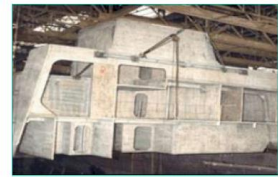
Superstructure Frigate La Fayette (1980 - 1990)
